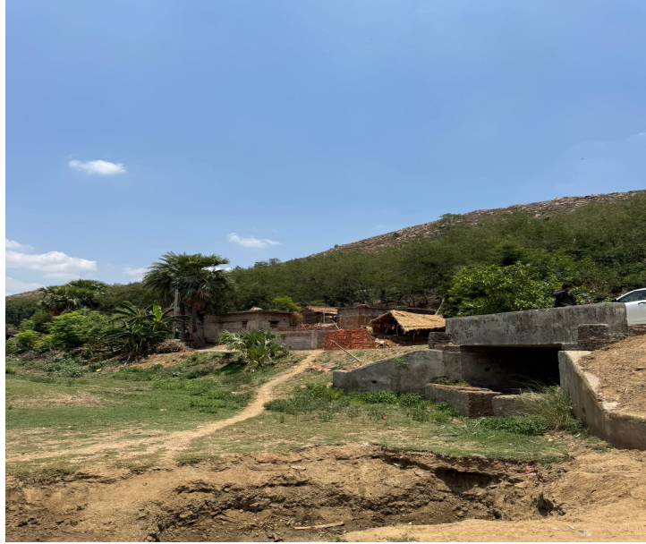
Figure 2: Rocky terrain and deep water tables make drilling difficult in Gaya.
